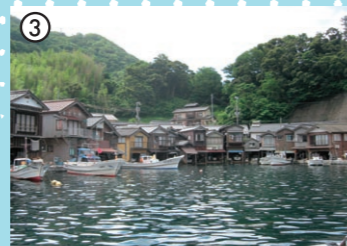
3 Ineura Funaya-gun, The boathouses of Bay (Ine Town) The street is lined with funaya houses. Their first floor is the storage space and their boat workshop, and the second floor is their living space.
